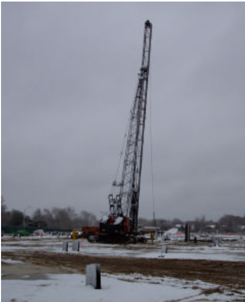
Photo 9: November 13, 2004 – pile driving equipment
