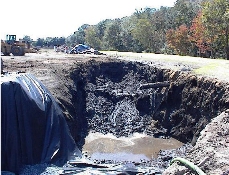
September 3, 2004 – View of the North Corridor facing South showing “Outlet 1”.
