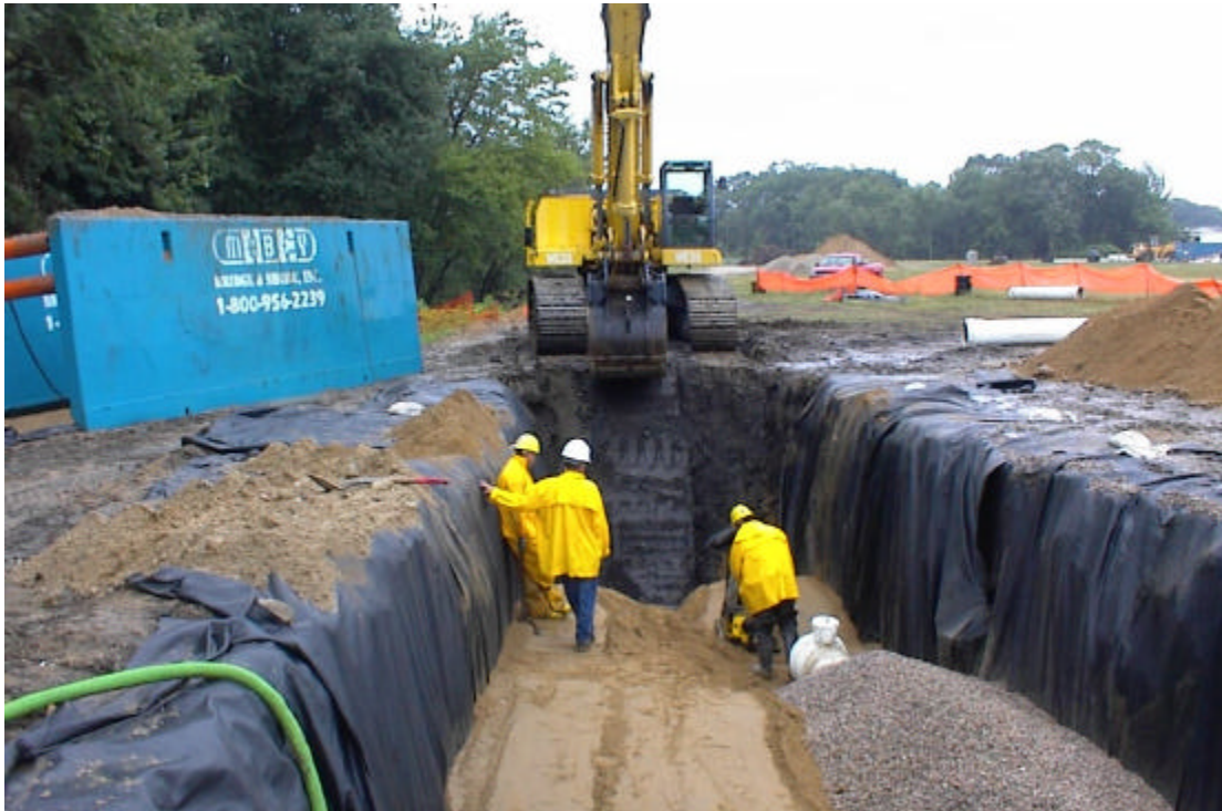
July 13 & 19, 2004 - Continued excavation and utility installation along south utility corridor.
