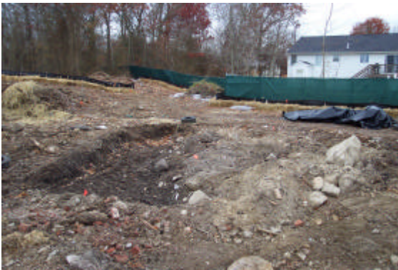
Photo 5: November 11, 2004 – north stockpile 8 facing northwest
