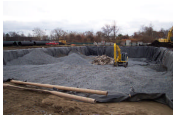
Photo 4: November 11, 2004 – south detention basin facing southwest
