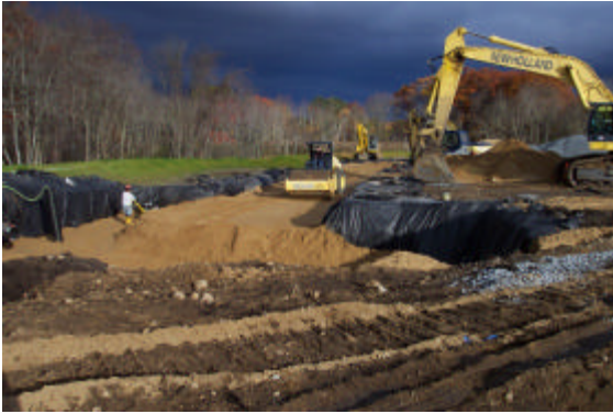
Photo 1: November 3, 2004 - north gross excavation area
