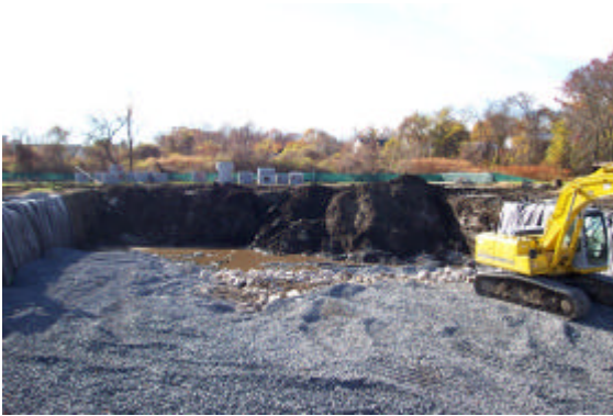
Photo 3: November 8, 2004 – south detention basin facing south
