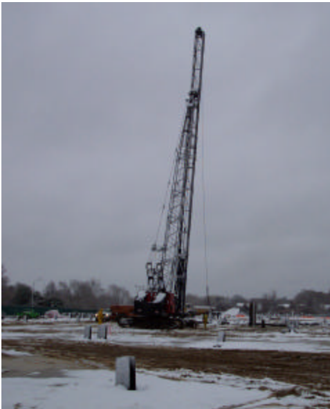
Photo 9: November 13, 2004 – pile driving equipment
