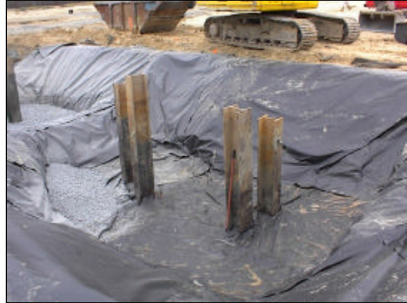
Photo 8: December 6, 2004 – Pile cap excavation, lined prior to backfill, facing northeast.
