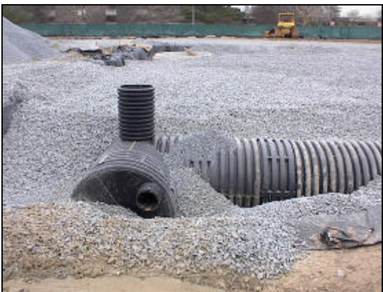
Photo 5: December 6, 2004 – South detention basin construction, facing east.
