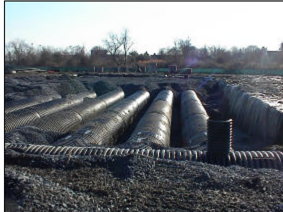
Photo 4: December 3, 2004 – South detention basin construction, facing south.
