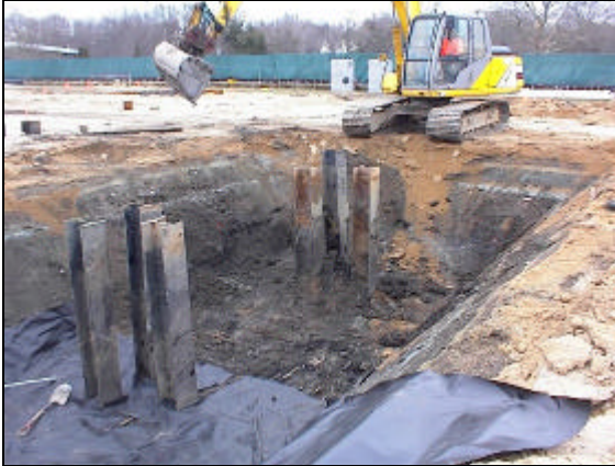
Photo 7: December 6, 2004 – Pile cap excavation, closer view, facing northeast.
