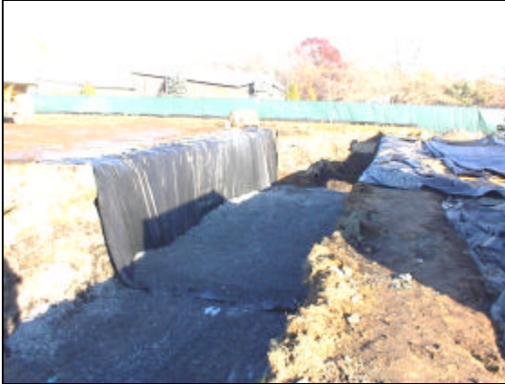
Photo 1: November 17, 2004 – North detention basin excavation area, photo facing east.
