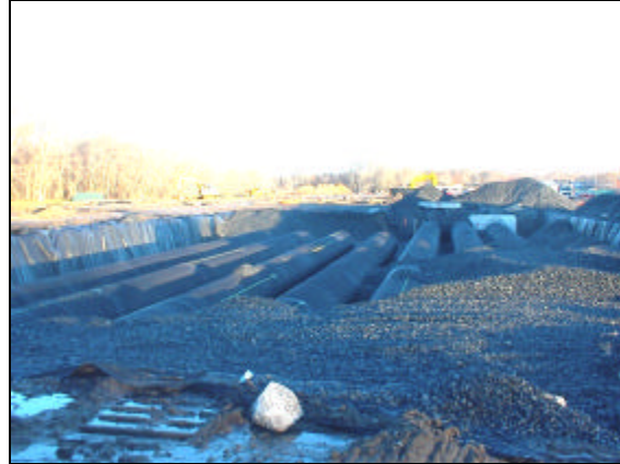
Photo 2: November 29, 2004 – South detention basin construction, photo facing north.
