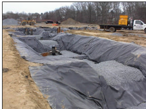
Photo 6: December 6, 2004 – Building footprint pile cap and grade beam excavations, facing southwest.
