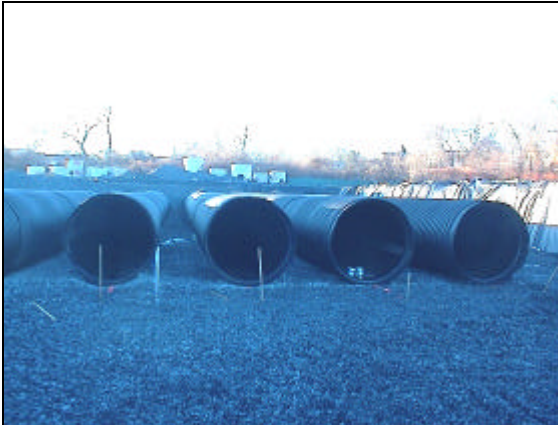
Photo 3: November 29, 2004 – South detention basin construction, photo facing south.
