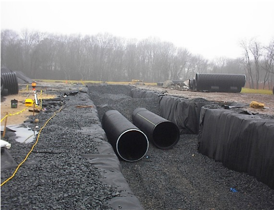
Photo 3: North Detention Basin pipe installation and gravel backfilling (facing west-northwest).
