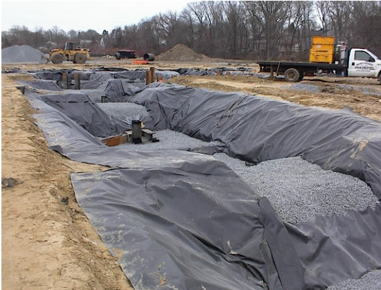
Photo 7: Partially completed row of pile caps (facing south-southwest).
