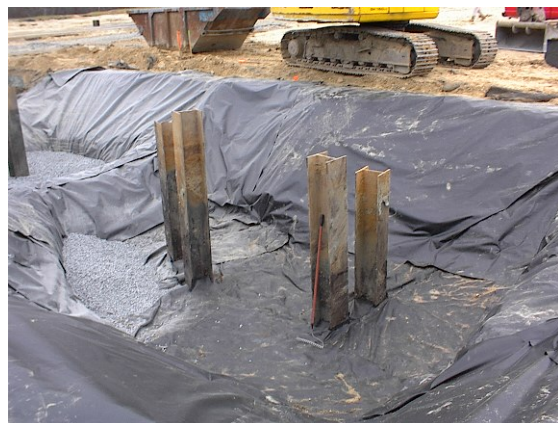
Photo 6: Typical geotextile fabric barrier placed in excavated pile cap area.
