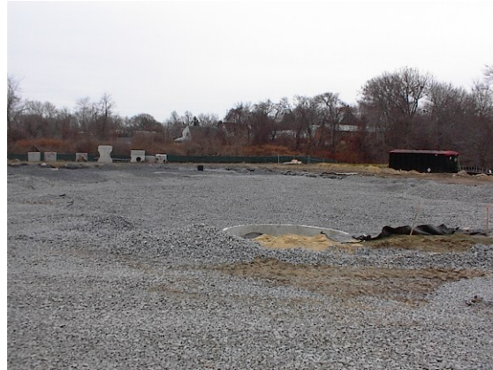
Photo 2: South Detention Basin after completion of gravel backfill (facing south-southwest).
