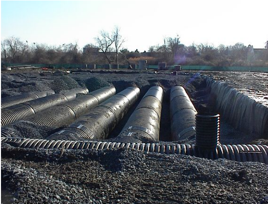
Photo 1: South Detention Basin during gravel backfill (facing South).
