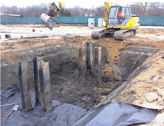
Photo 5: Typical excavation of pile cap.
