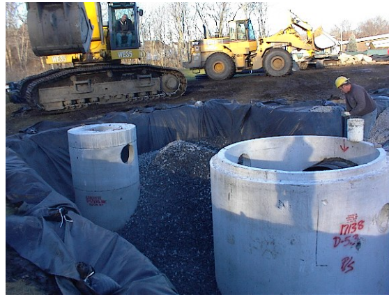
Photo 4: North Detention Basin catch basin and manhole (typical).
