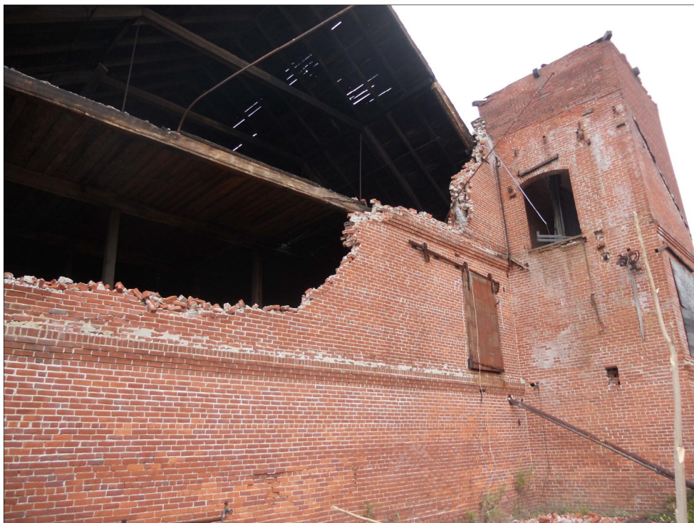
Unsupported Partially Collapsed Brick Wall
