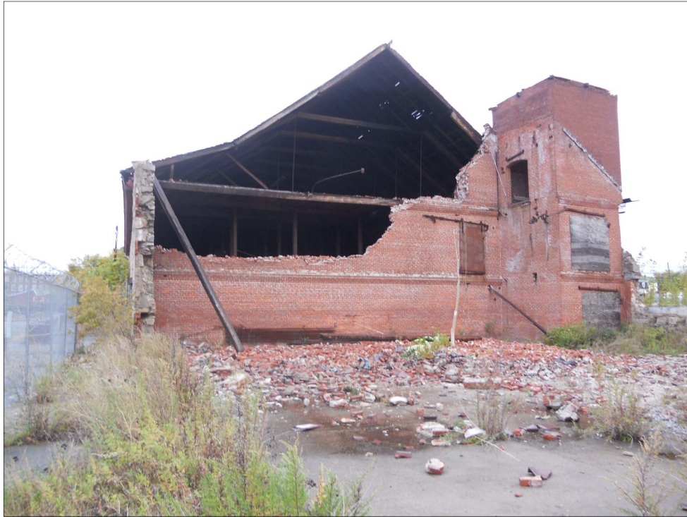
East Building Elevation of Partially Collapsed Brick Wall
