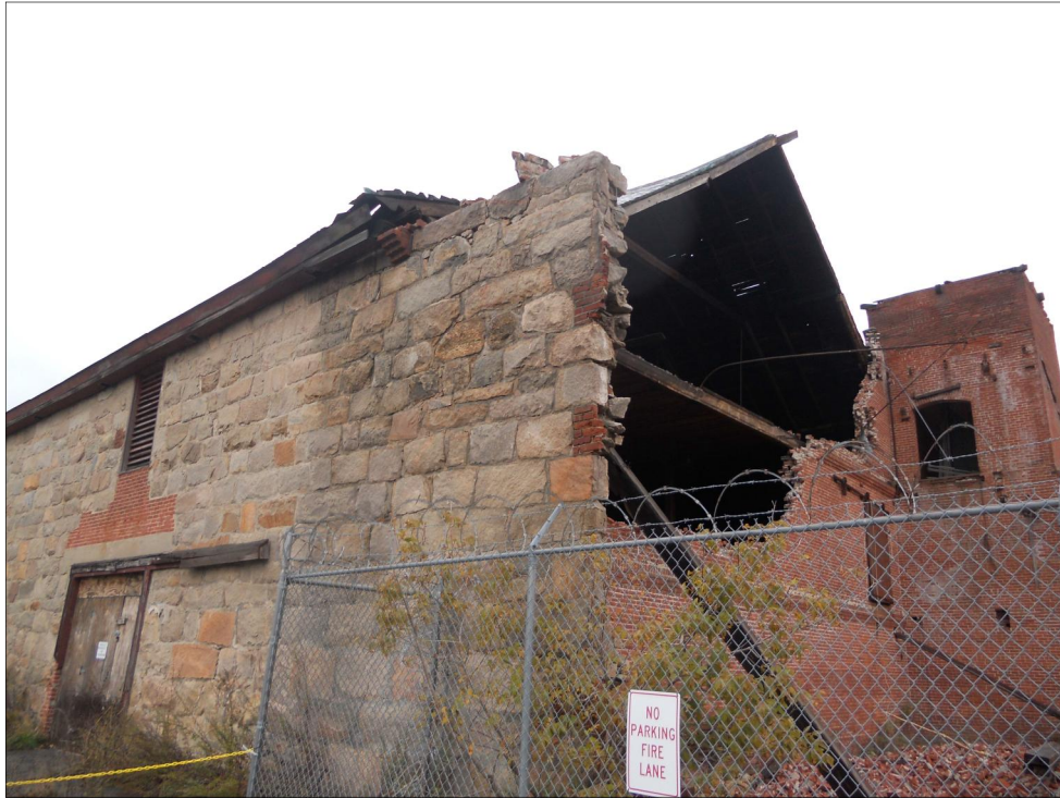
Unsupported Masonry Wall & Roof Truss Connection
