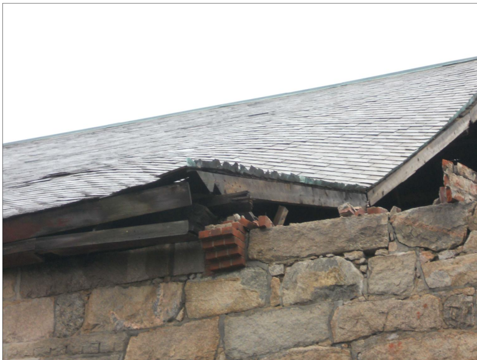
Failed Roof Truss Connection at Partially Collapsed Brick Wall
