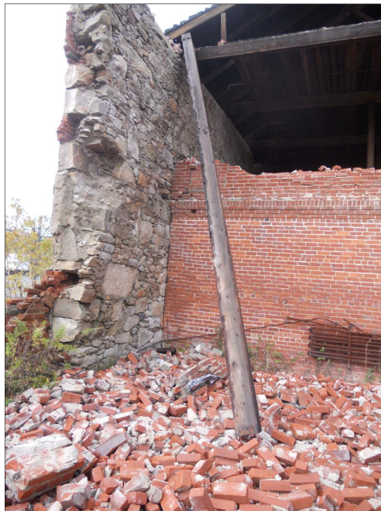
Dislodged Roof Truss Lower Chord
