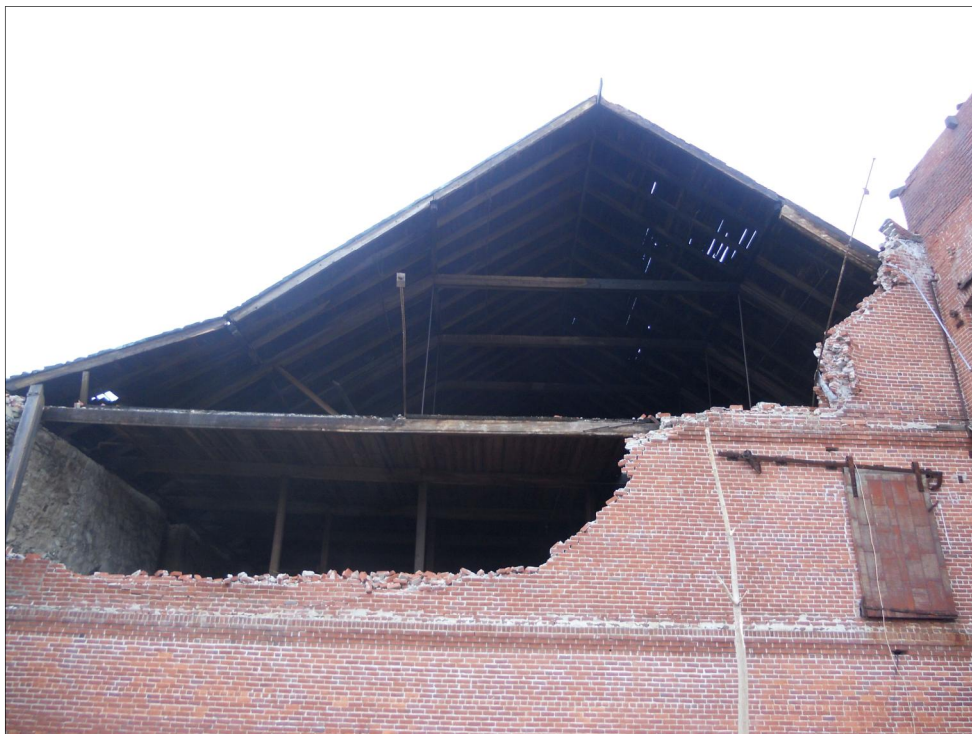
Roof Truss Failure
