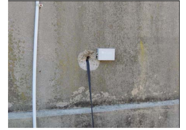
REFURBISH EXISTING ELECTRICAL & COMMUNICATION WIRING TO ATTAIN FLOOD-PROOF CONDITION. (PENDING)
