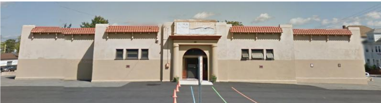
West Façade- Madeira Avenue Entrance
