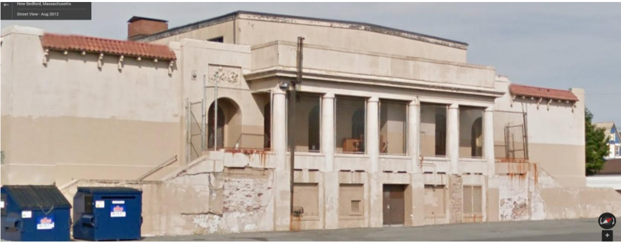
East Façade-Belleville Ave.
